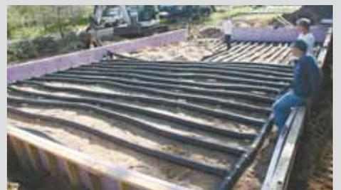
He laid one layer of heat tubes over the insulation. They were covered with sand, then a second layer of tubes was laid perpendicular to the first.
