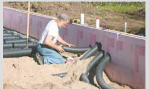
An in-line fan is used to push/pull air through the closed system of 4-in. corrugated drain tiles.
