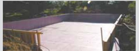
Staus prepared the base for the greenhouse by excavating 4 ft. of soil and laying down 2-in. rigid Styrofoam panels.
