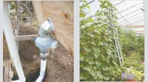
Twin 4 by 10-ft. solar thermal collectors help to heat the 30 by 72-ft. FarmTek high tunnel. Hot air is piped through an insulated sand base under the greenhouse.
