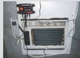
Mark Wittman uses a CoolBot micro-controller to monitor his walk-in cooler. It adjusts an air conditioner fan and compressors as needed to keep the cooler at the desired temperature.
