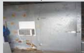
Mark Wittman uses a CoolBot micro-controller to monitor his walk-in cooler. It adjusts an air conditioner fan and compressors as needed to keep the cooler at the desired temperature.
