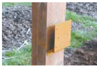
Bracket is made from 16-ga. steel and mounts onto upright posts with 2 screws.
