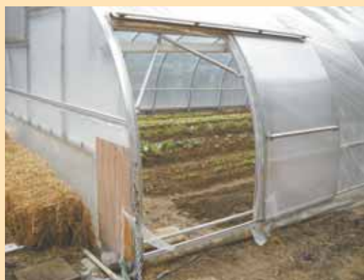
Phil Norris designed his rolling high tunnel greenhouse to traverse four 48-ft. plots over the course of the growing season.
