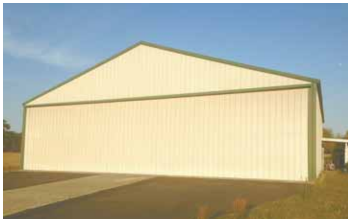
Kin Purvis needed a door for the 50-ft. wide opening on his airplane hangar, so he and his friend built a one-piece unit that provides plenty of clearance.
