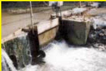
Small Creek Power Generator (Page 19)
