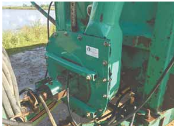
Photo shows pump and bearing housing after installation.
