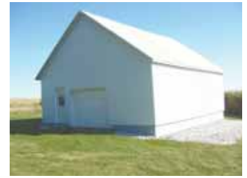
Howard Reischauer converted an old corn crib into a 30 by 32-ft. farm shop. He covered the exterior with steel siding and installed overhead garage doors at both ends.
