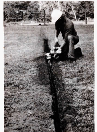
Trencher digs 2½ in. wide trench for burying pipe or cable.
