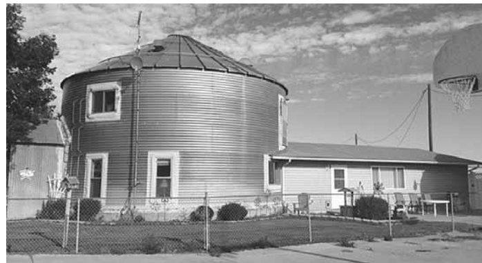
Kendell and Cindy Karlson’s converted bin has one special feature not found in most houses - a fireman’s ladder between the second floor and cone section loft.
