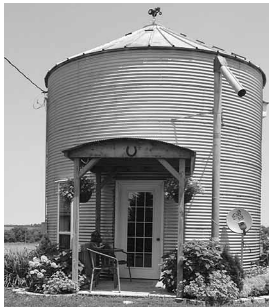
Donna Thieme of Humphreys, Mo., turned an 18-ft. dia. bin on her property into this B&B. A space-saving staircase wraps around the inside of bin’s east side.
