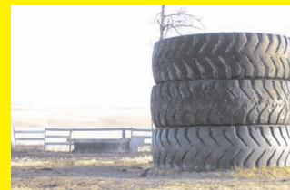
Big Tire Water Storage Tank (Page 28)
