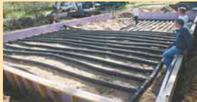
Greenhouse Built On Solar Heat Pipes (Page 3)
