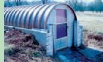
Greenhouse Built From Fiberglass Tank (Page 18)
