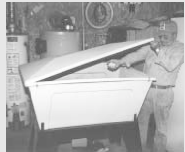
Corn-burning furnace and 14-bu. metal hopper are housed in a mud room that Foster built onto his house.
