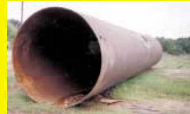
Big Culvert Made From Tank Car (Page 9)
