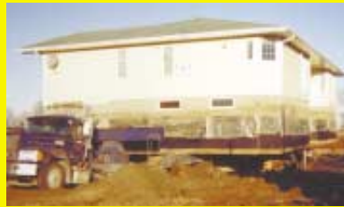
Moving Houses With Basement On (Page 2)
