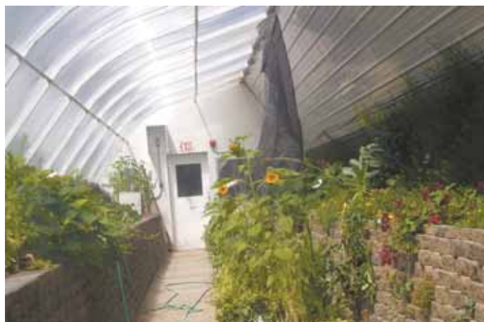
Greenhouse is buried 5 ft. below ground. There are now 17 full-size units in place across 6 states and Canadian provinces.
