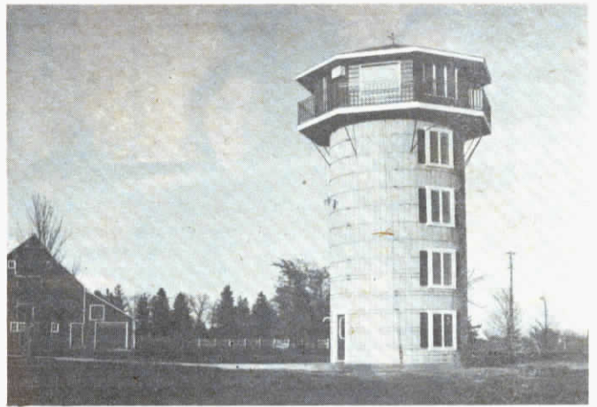
The 35-ft. tall silo house contains 1600 sq. ft. of living space.
