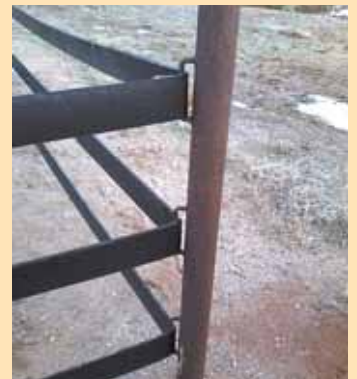
Belt is threaded through retainers at each pipe until it reaches opposing end post.
