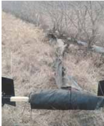
Operator drives skid loader ahead as spindle winds up fabric.
