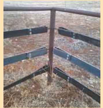
Belt tension device uses a threaded rod that runs through a pipe sized to match the width of belt being used. Threaded rod is welded to corral's corner post.
