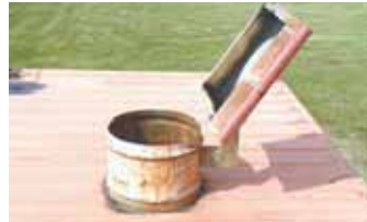
He cut a hole in container roof for access and then cut a 35-gal. drum in half and set it over hole, adding a hinged lid (left). Container's shale pad prevented locking rods on door from engaging so he shortened the rods slightly.
