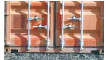
He cut a hole in container roof for access and then cut a 35-gal. drum in half and set it over hole, adding a hinged lid (left). Container's shale pad prevented locking rods on door from engaging so he shortened the rods slightly.
