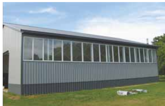
When Nelson Brubaker built this big 50 by 64-ft. shop building, he bought 19 used kitchen patio doors and installed them in a row along the entire south side of the building, just underneath a 2-ft. overhang.
