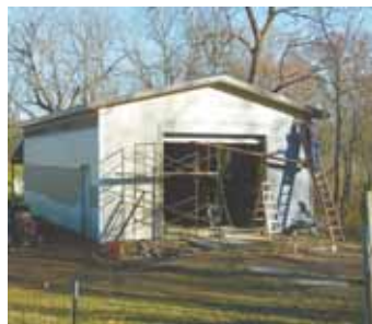
“For the building’s exterior, I picked up fiber cement siding at a farm sale for pennies on the dollar,” says Eby.
