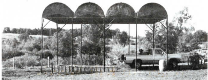
Shed holds 144 round bales and 848 small square bales of straw (top). Tank sections are mounted on framework built out of heavy wall oil field pipe (bottom).
