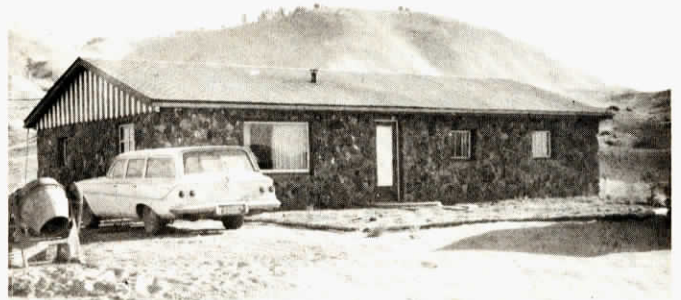
Louis and Sharon Watson used 18 pickup loads of rocks to build their 3-bedroom home, shown above.
