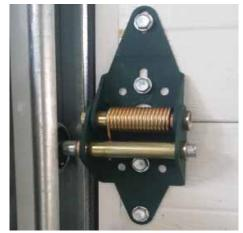
Spring-loaded garage door hinge pushes door gap shut to keep heat from leaking outside.
