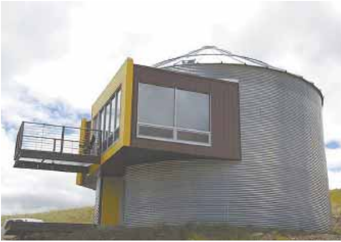
Two-story grain bin home has “bump outs” painted bright gold/yellow to match the original MFS logo still on the corrugated bin. A 7-ft. steel deck with bar grate flooring is just outside the living room.
