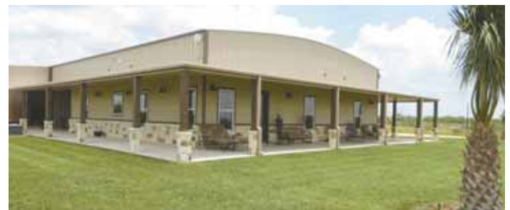
“Barndominiums” are built on concrete slabs, with the walls and roof made of metal. Popular designs include a home and workshop or garage connected by a breezeway.
