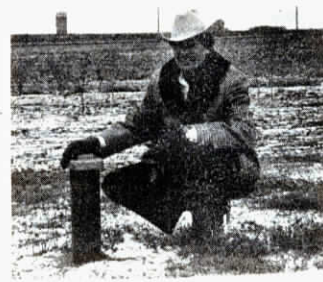
The only visible part of the Pollert’s well is a capped pipe. Pollert, shown above, says the two wells (48-ft. deep) cost $1,724 for drilling and plumbing, and the heat pump cost $3,540 installed.
