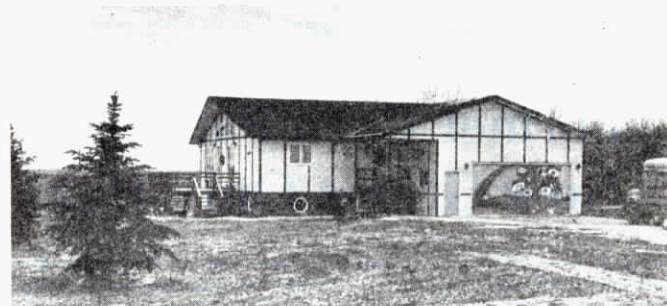
Pollert’s ground-water furnace not only heats the house in the winter but cools it in the summer.
