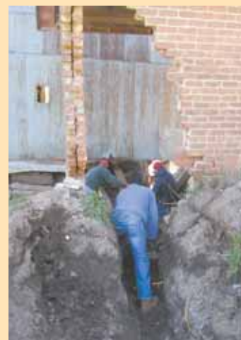
Bob and Janet Nelson are working to completely restore the elevator with help from friends, family, and contractors. A house-moving company lifted the entire building with steel beams so the foundation could be rebuilt.
