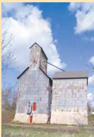
Bob and Janet Nelson are working to completely restore the elevator with help from friends, family, and contractors. A house-moving company lifted the entire building with steel beams so the foundation could be rebuilt.
