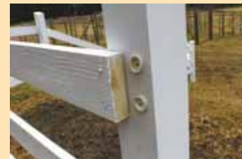
Top 1 ft. of concrete footing forms a “half-lap”. A short length of PEX tubing inserted part way up lap is used to insert a bolt (left). Thin pvc pipe rings behind boards serve as spacers to keep water from collecting.
