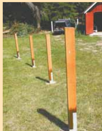
Hybrid fence posts are made from wood set in 4-ft. long concrete footings. “With this design I don’t think I’ll ever have to rebuild,” says Eric Little.
