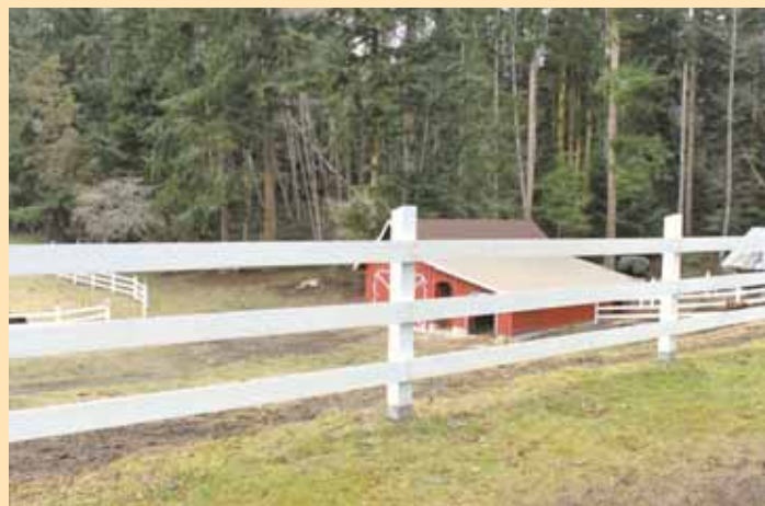
Wood part of post stands 5 in. above ground, with about 32 in. of the concrete footing buried.
