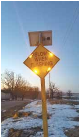
When solar-powered sign senses anything moving past it at less than a preset speed, it flashes for 3 min. to warn faster drivers to slow down.
