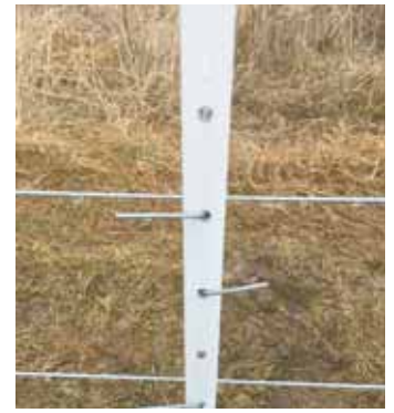
Fiberglass posts are pre-drilled with holes every 2 in., making it easy to attach high tensile wire that’s bent into a U-shape.
