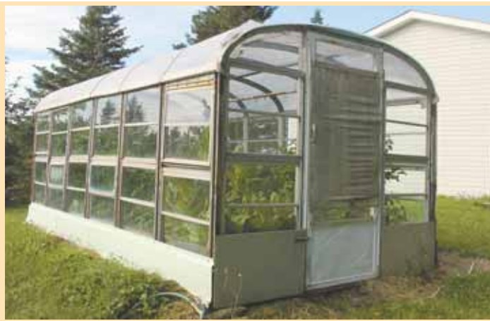
Harry Coates cut off the back half of a 72-passenger bus, removed the floor and used windows from front half of bus to give his greenhouse two sets of windows down each side.
