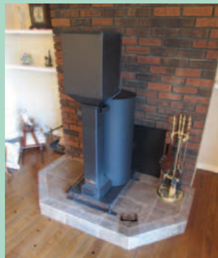
Liberator rocket heater installs like a conventional wood stove, but uses less fuel.
