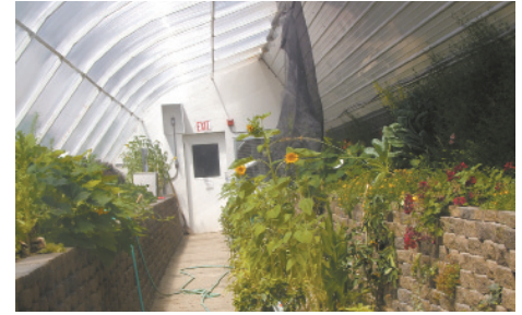
Greenhouse is buried 5 ft. below ground. There are now 17 full-size units in place across 6 states and Canadian provinces.
