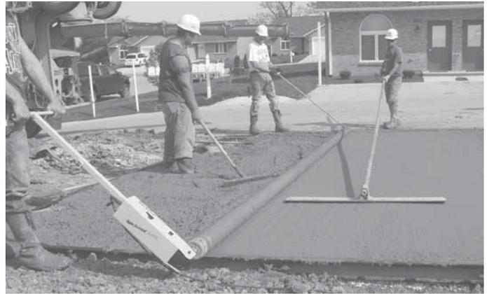
build drive-over curb and gutters and valley pans in a single pass.
