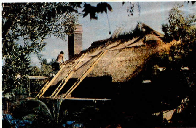
Finished thatched roofs are 12 in. thick, providing good insulation.
