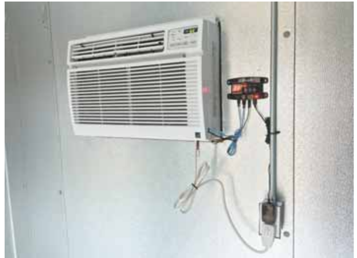
Controller comes with a ready-to-install LG window air conditioner capable of maintaining temperatures as low as 34°F.
