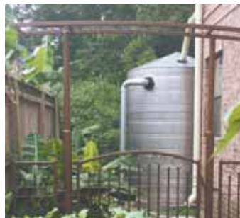
Stainless steel rain tanks are available in a variety of sizes. Photo shows pipes entering and exiting tank and also a diverter pipe.
