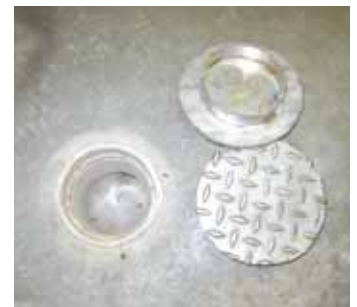
A metal cap is placed over each floor port when they're not being used.
