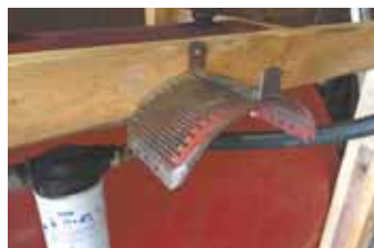
Pump hoses store neatly on brackets made from old combine parts.
