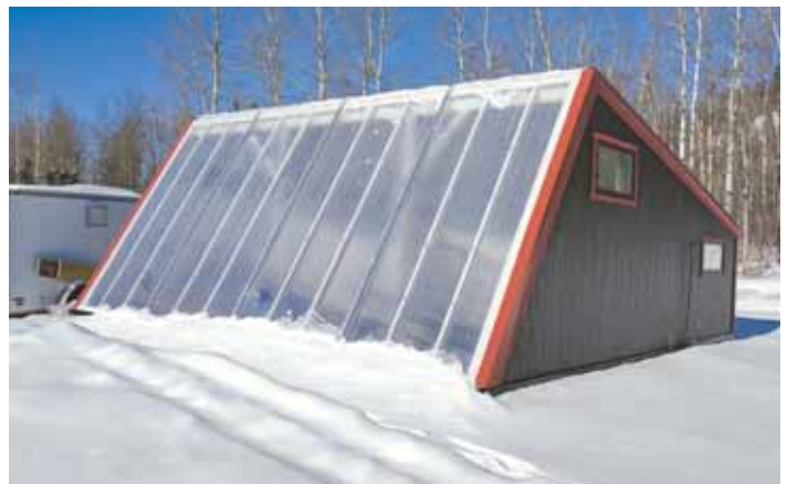
Greenhouse has a 4-ft. deep crushed rock bed beneath a sloped greenhouse wall. Warm air is pulled down into rock bed and a fan pulls the heat out into greenhouse.
