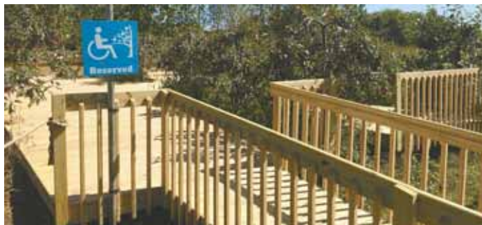
An H-shaped, 42-ft. long deck wraps around 18 Cortland apple trees. It lets people in wheelchairs pick apples.
