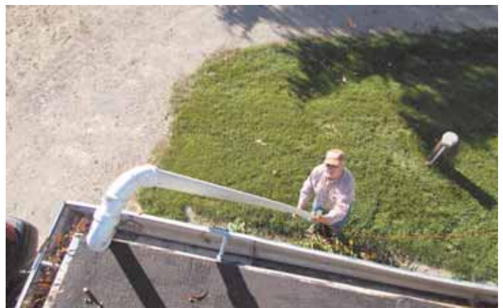
Bob Manzke points his pvc contraption at an angle to blow leaves out of his gutters.
