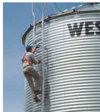
Grain bin fall protection system consists of a D-ring that slides along a cable next to ladder.
