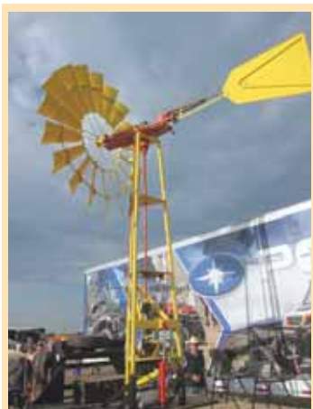
Phoenix windmill produces AC electricity. Fan assembly and tail drives a gearbox and driveline, which in turn chain-drives a generator.
