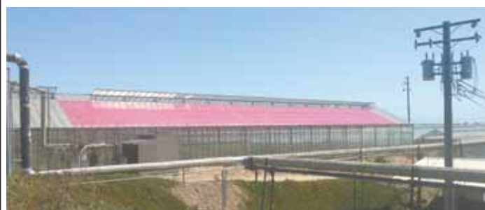
This greenhouse is covered with LUMO solar panels to boost plant growth and also generate electricity. Panels convert green light to red light, the most efficient light for photosynthesis.
