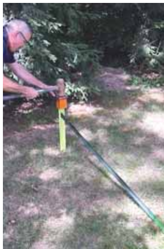
T-post fits into U-shaped metal base with 3 holes on each side. A bolt inserted through lower set of holes serves as a hinge point. You hammer base into ground, then insert a wooden dowel through upper set of holes to keep post upright.
