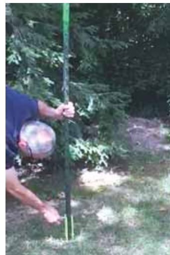
T-post fits into U-shaped metal base with 3 holes on each side. A bolt inserted through lower set of holes serves as a hinge point. You hammer base into ground, then insert a wooden dowel through upper set of holes to keep post upright.
