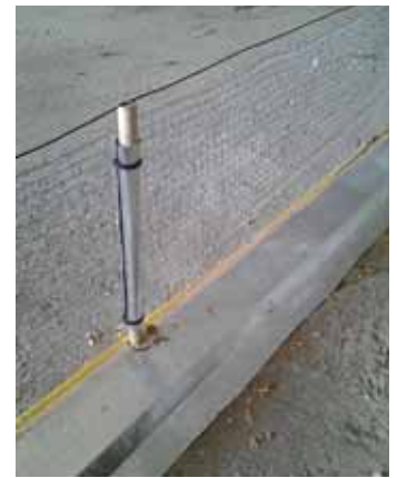
An electric fence charger hooks up to 1-ft. tall wire fence that's mounted on a 2 by 4 base covered by metal flashing.
