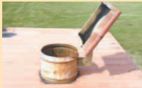
He cut a hole in container roof for access and then cut a 35-gal. drum in half and set it over hole, adding a hinged lid (left). Container’s shale pad prevented locking rods on door from engaging so he shortened the rods slightly.
