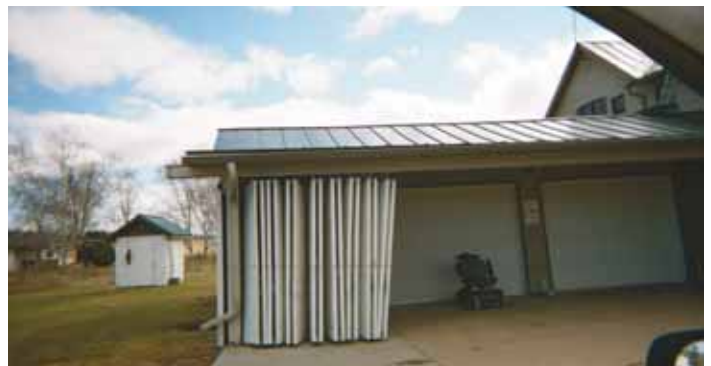
Orville Krueger attached a bunch of used overhead garage doors together across the front side of his 30-ft. wide carport, hanging them vertically from a track. Doors are hinged together in such a way that they open and close accordion-style.
