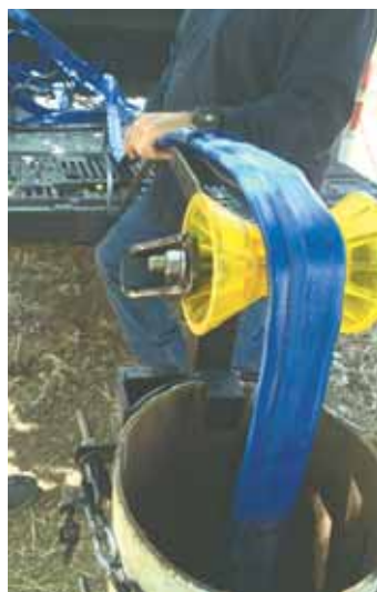
To install WellHose DIY Drop Pipe, you just attach a pump to end of hose and lower it into well. Hose's smooth fabric results in energy savings and less head loss.
