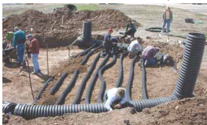
Climate Battery blows hot, humid air through pipes and into the cool soil beneath a greenhouse, where heat and humidity are released. By the time the air returns to the greenhouse it's cooler and drier.
